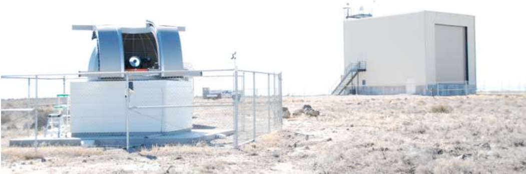
Figure 22: LIDAR and BRFD station (right building).
