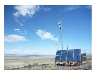
Figure 3.40: The Black Rock Mesa communication tower, one of three in the array. There are there stands each with solar panels. Those stands contain batteries, data acquisition PC and network instruments for long distance link.
