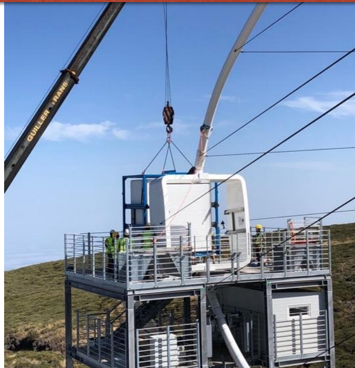
Camera Installation On the telescope
