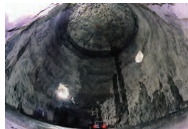
Completion of excavation a large cavity with 40m in diameter and 58m in height Construction of a stainless tank by attaching stainless plates on the wall of the cavity 直径40m 高さ58m の巨大空洞が完成 この後空洞の壁面にステンレス板が取り付けられた
