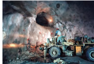
Excavating hard rock, Hida gneiss, using a blasting method 飛驒片麻岩の硬い岩盤を掘り進む掘削作業
