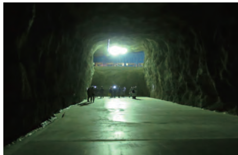
Figure 3: The new Hall G in the Kamioka mine. About 12 kilotons of rock were removed to make room for the new Gd-capable water systems.
