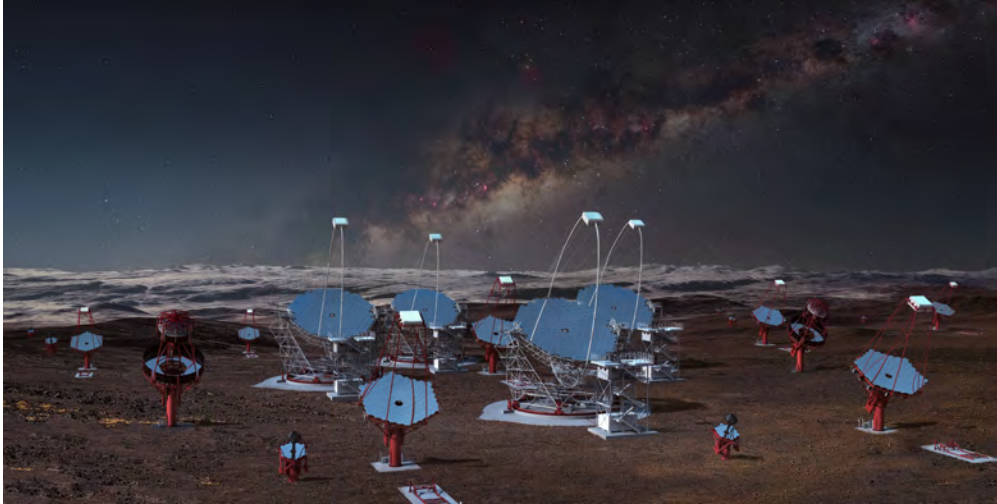
Fig. 1. Artist view of the CTA observatory. CTA consists of three types of telescopes, Large Size Telescopes (23 m diameter), Mid Size Telescopes (12 m) and Small Size Telescopes (4 m), and covers the broad energy band from 20 GeV to 300 TeV. [Credit: Gabriel Pérez Diaz (IAC)/Marc-André Besel (CTAO)/ESO/ N. Risinger (skysurvey.org)]
