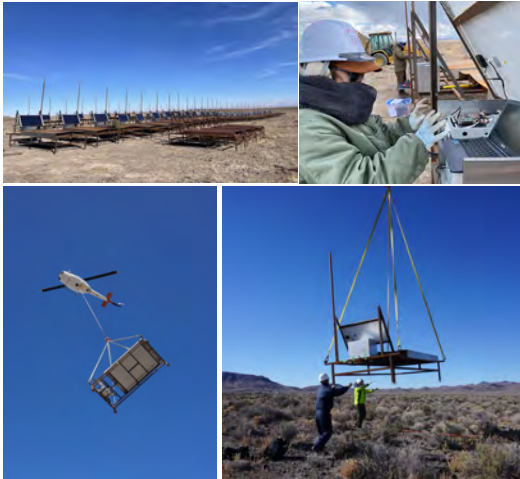
Fig. 22. Photographs of detectors being installed for the TALE infill experiment, taken in October 2022. Once the SDs were moved to the staging area (upper-left), they were finally confirmed to be in normal operation there (upper-right). Each SD was then transported by helicopter to a pre-determined installation point (lower).
