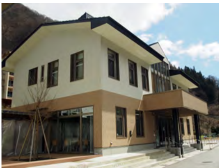
Fig. 1. Surface Research Building.
