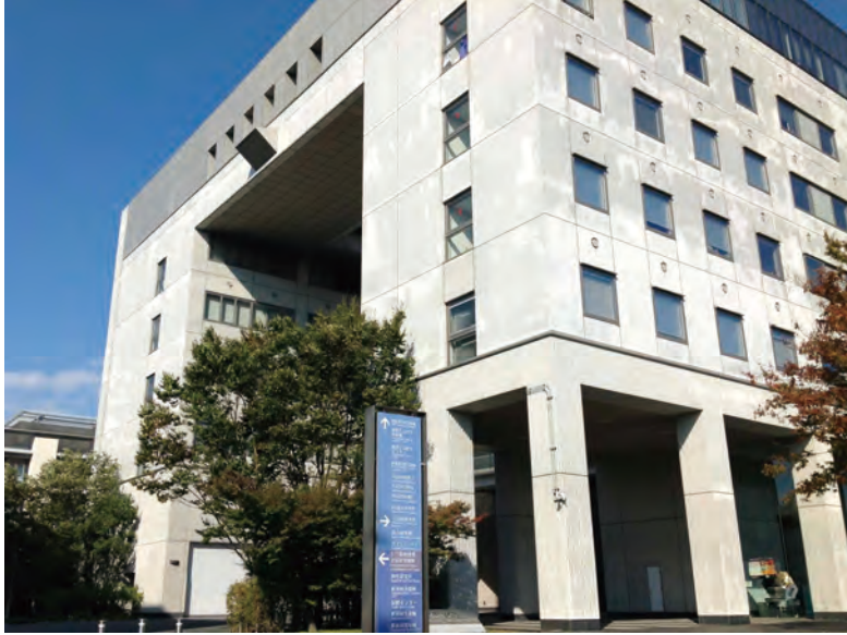
The ICRR building at Kashiwa, Chiba, Japan.
