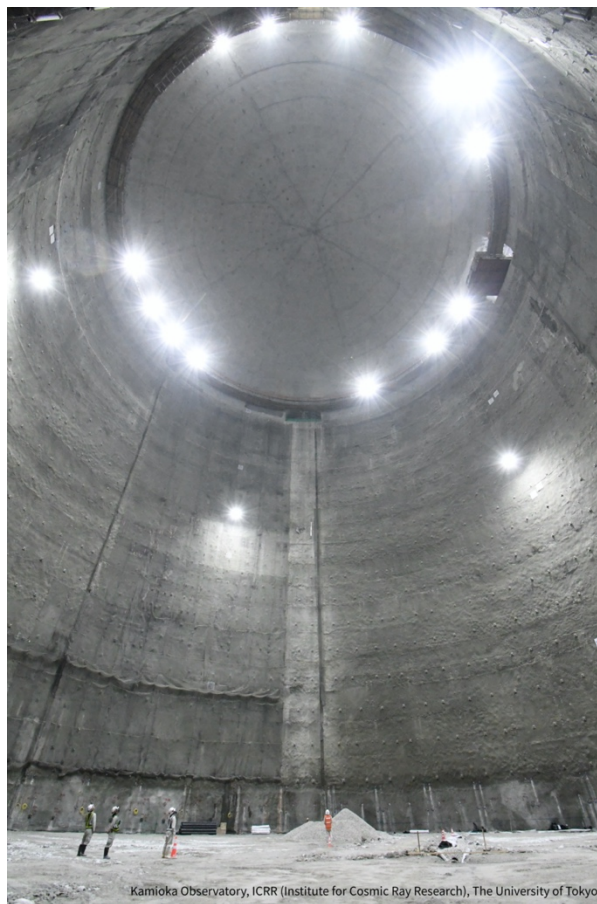
The main Hyper-Kamiokande cavern after excavation completed
