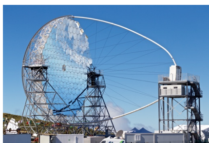
Figure 1: Completed LST1 in La Palma in October 2018.
