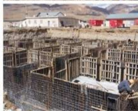
MD construction scene
