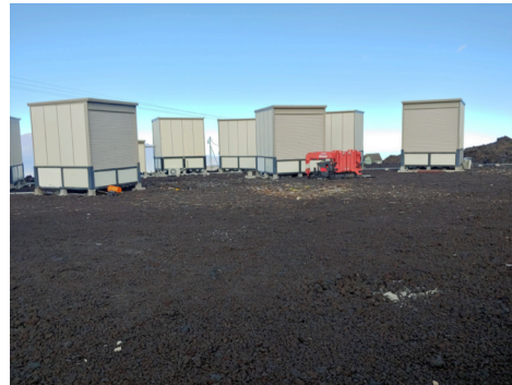
Fig.4: View of the Mauna Loa site after cleaning up the debris.
