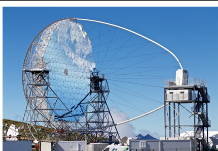
Figure 1: Completed LST1 in La Palma in October 2018.
