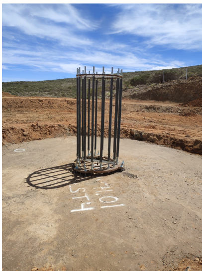
Figure 5: cage of the central pin of LST-2
