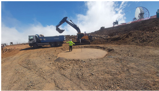
Figure 4: LST4 status of construction works
