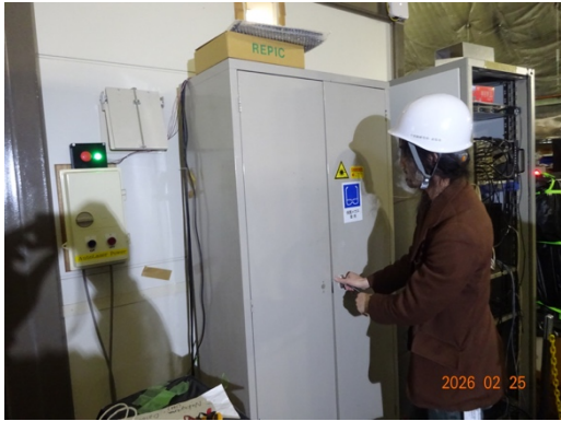
Figure 2: OD laser cabinet. A green LED lamp is on during the operation. This is off if the cabinet door is open.
