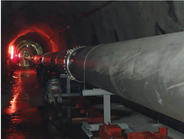
Fig. 7. 3-km beam tube in the Y-arm tunnel.
