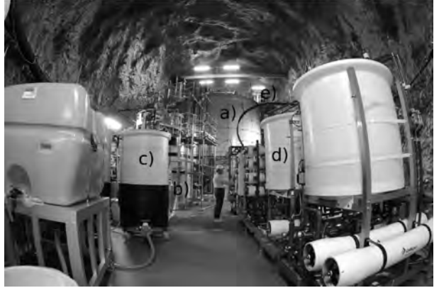
Fig. 21. In the new cavern the Gd pre-mixing and pre-treatment 15 ton tank (front left), the selective filtration system (front right) and the 200 ton tank (rear of the hall) have been installed.
