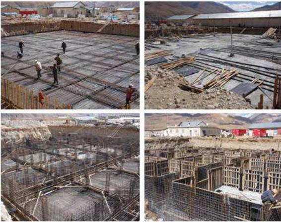
Fig. 9. Construction scene of underground muon detectors in 2010.
