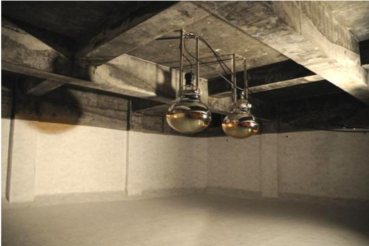
Tyvek sheet walls and two 20 inch PMTs
