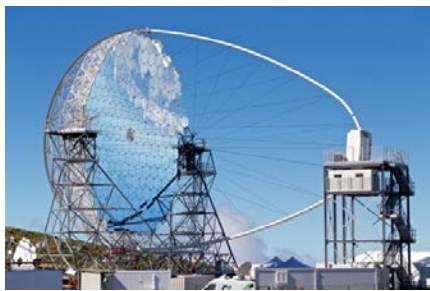
Figure 1: Completed LST1 in La Palma in October 2018.
