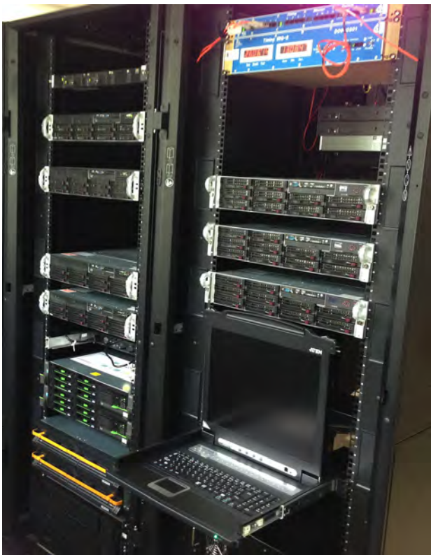
Fig. 8. Part of DAQ system for KAGRA. All data from KAGRA is collected into these computers. The DAQ system and real time front-end computers are synchronized by timing system shown in blue chassis in this picture.
