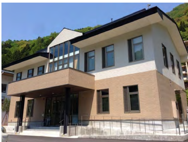
Fig. 2. Data acquisition & analysis building for KAGRA
