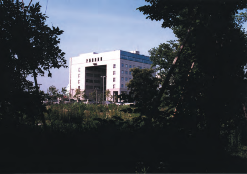
The ICRR building at Kashiwa, Chiba, Japan.
