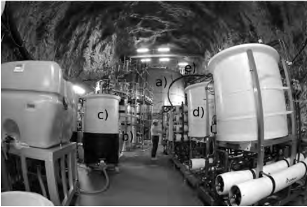
Fig. 19. In the new cavern the Gd pre-mixing and pre-treatment 15 ton tank (front left), the selective filtration system (front right) and the 200 ton tank (rear of the hall) have been installed.
