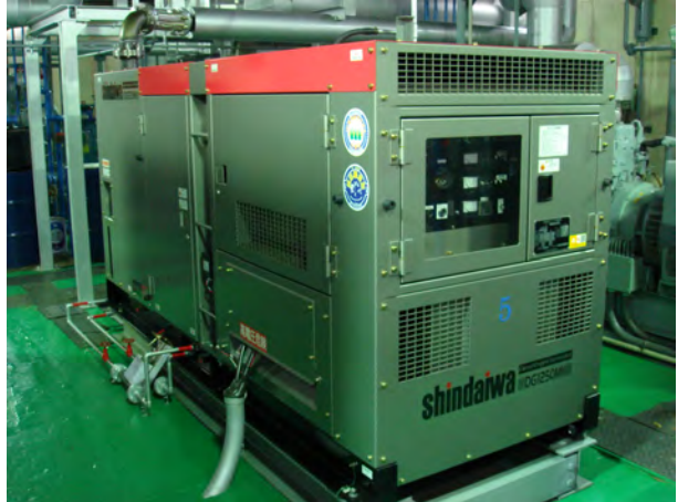
Fig. 2. A dynamo of 115KV.
