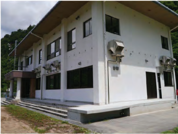
Fig. 2. Refurbished Hokubu Kaikan for Kamioka branch of GWPO
