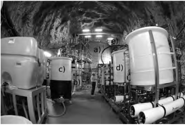
Fig. 18. In the new cavern the Gd pre-mixing and pre-treatment 15 ton tank (front left), the selective filtration system (front right) and the 200 ton tank (rear of the hall) have been installed.
