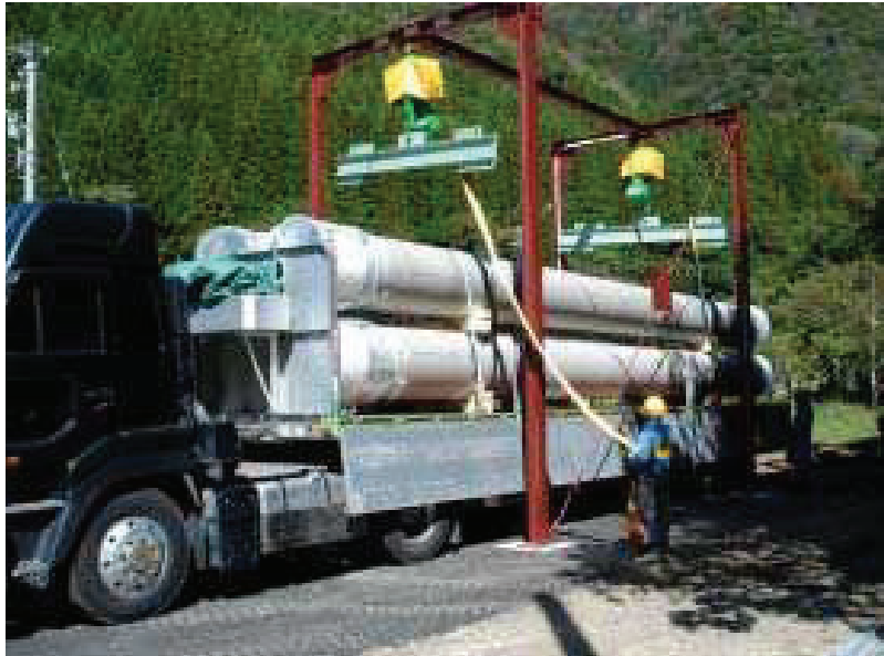
Fig. 7. Tube delivery to the storage tunnel.
