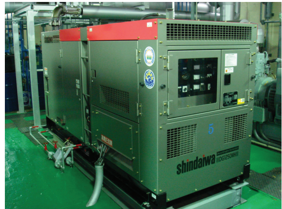
Fig. 2. A dynamo of 115KV.
