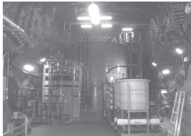
Fig. 3. In the new cavern the Gd pre-mixing and pre-treatment 15 ton tank (front left), the selective filtration system (front right) and the 200 ton tank (rear of the hall) have been installed.
