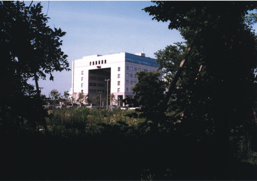
The ICRR building at Kashiwa, Chiba, Japan.
