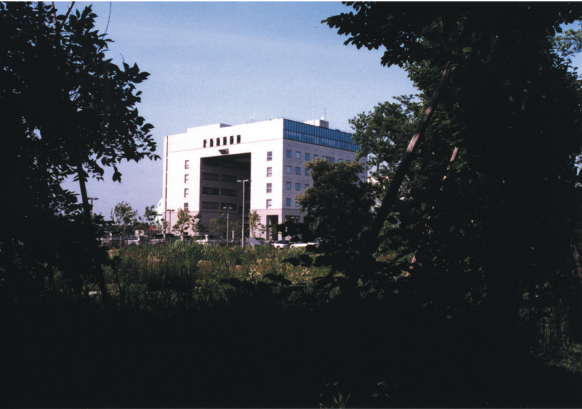
The ICRR building at Kashiwa, Chiba, Japan.
