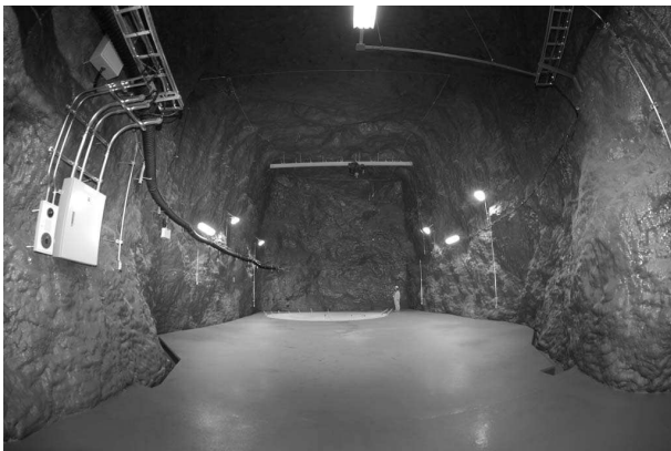
Fig. 2. A new cavern was excavated for the R&D study of the gadolinium project in 2009. The size of the cavern is 10 m wide, 15 m long, 8~10 m high. A 200-ton water tank and a water purification system will be installed in 2010.
