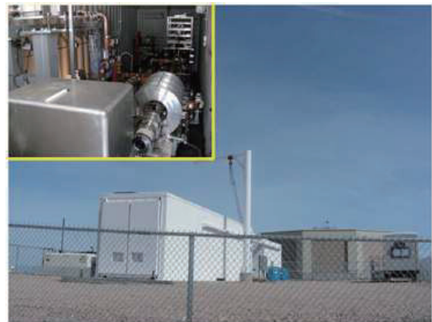
Fig. 1. The TA-LINAC that was installed in the BRM site. The accelerator part is in a 40-ft container, which is located 100 m in front of the fluorescence station. The photo of the accelerator taken from the electron-gun side is also shown.
