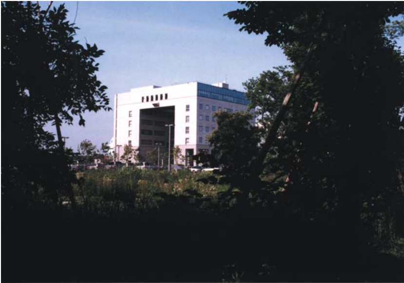
The ICRR building at Kashiwa, Chiba, Japan.
