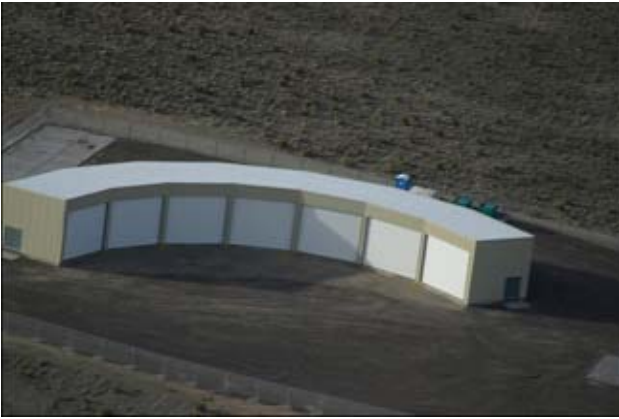
Fig. 11. The Middle Drum Observatory Building.
