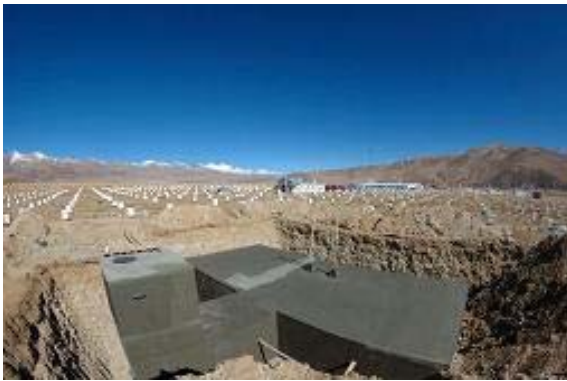
Fig. 7. Prototype muon detector viewed from outside, just before being covered with soil.
