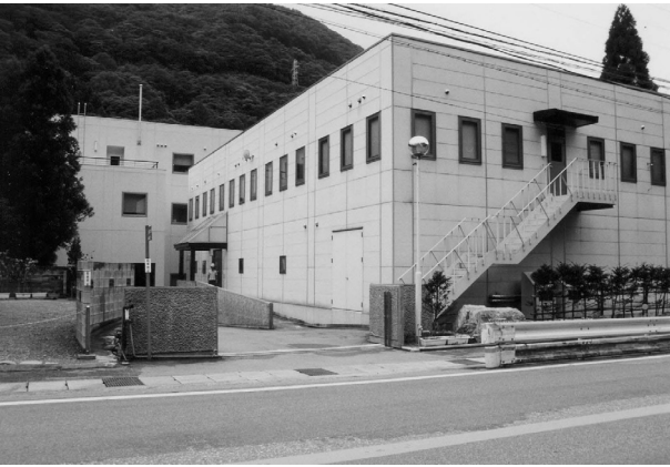
Fig. 5. Research offices and computer facility.
