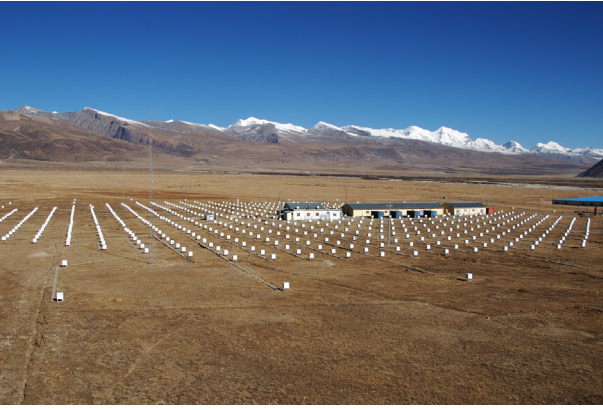
Fig. 2. 37000 m^2 Tibet-III array operating at Yangbajing.
