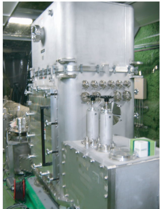
Fig. 16. This cryostat was installed in 2004 and its cryogenic test has been successfully finished. One-arm of the vacuum system was constructed and vacuum chambers for the input optics were fully installed.
