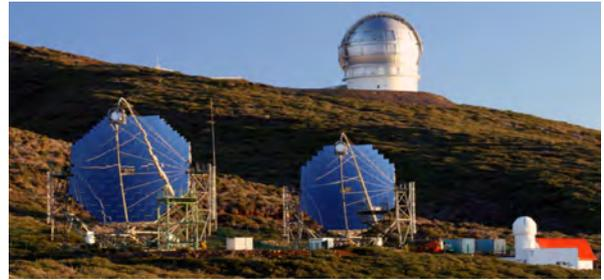
Fig. 6. MAGIC Stereo System with two Cherenkov telescopes of 17m diameters, so far achieved the threshold energy of 25GeV. It locates near the mountain top of the Roque de los Muchachos on the Canary Island of La Palma. Two telescopes are located with the distance of 85 meters.
