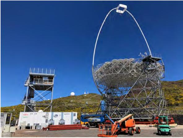
Fig. 5. The Large Size Telescope prototype (LST-1) under construction at Observatory de Roque de los Muchachos. The diameter of dish and mirror surface area are 23m and 400m<sup>2</sup>.
