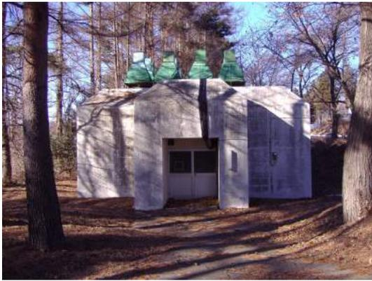
Fig. 3. One of the muon detector housings with concrete shielding.
