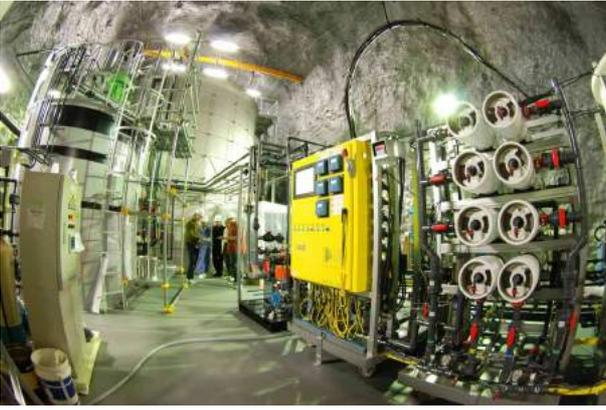
Fig. 23. In the new cavern the Gd pre-mixing and pre-treatment 15 m<sup>3</sup> tank (front left), the selective filtration system (front right) and the 200 m<sup>3</sup> tank (rear of the hall) have been installed.
