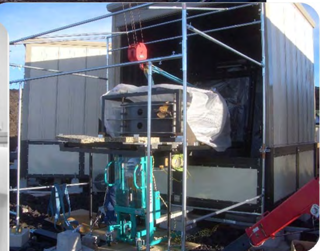
Installation of PLIs
