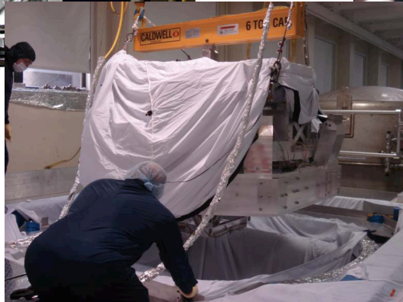
April 2008 – Quad-ISI BSC installation
