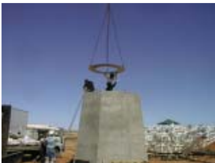
Setting the top plate on the telescope pedestal (Feb.'02)
