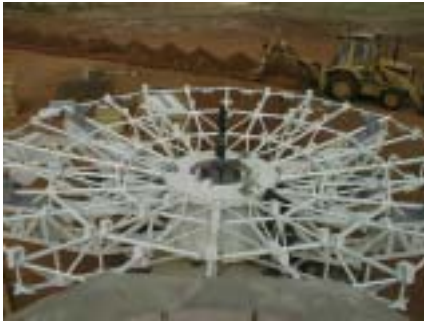
Assembly of the backing structure (Feb.'02)
