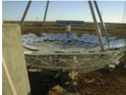
Setting small spherical mirrors (Mar.'02)
