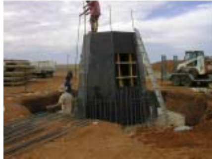
Formwork for the telescope pedestal base (Feb.'02)
