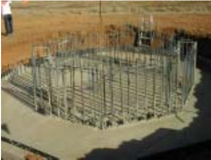
Construction of the telescope pedestal base (Jan.'02)
