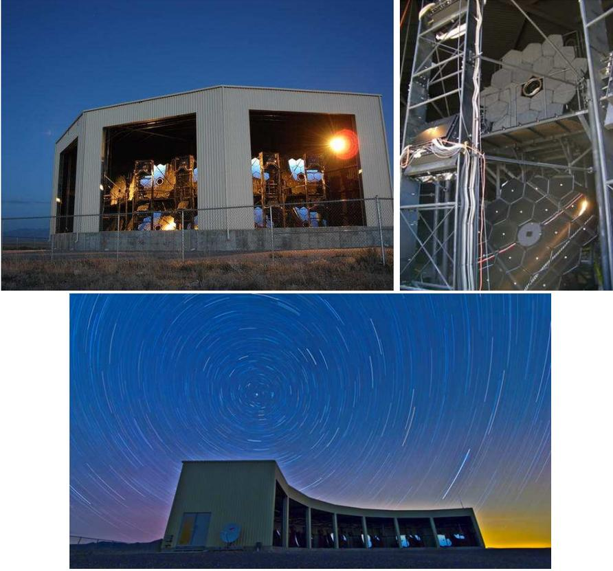
Figure 3.2: The BRM station (top-left), the fluorescence detectors of BRM station (top-right) and the MD station and MD fluorescence detectors transported from HiRes-I and HiRes II experiment (down).
