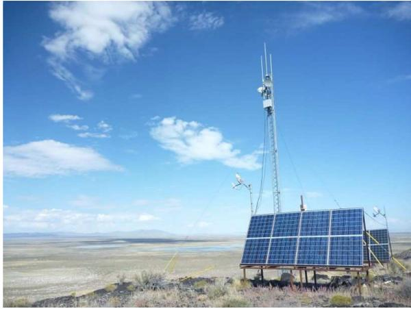
Figure 3.40: The Black Rock Mesa communication tower, one of three in the array. There are three stands each with solar panels. Those stands contain batteries, data acquisition PC and network instruments for long distance link.
