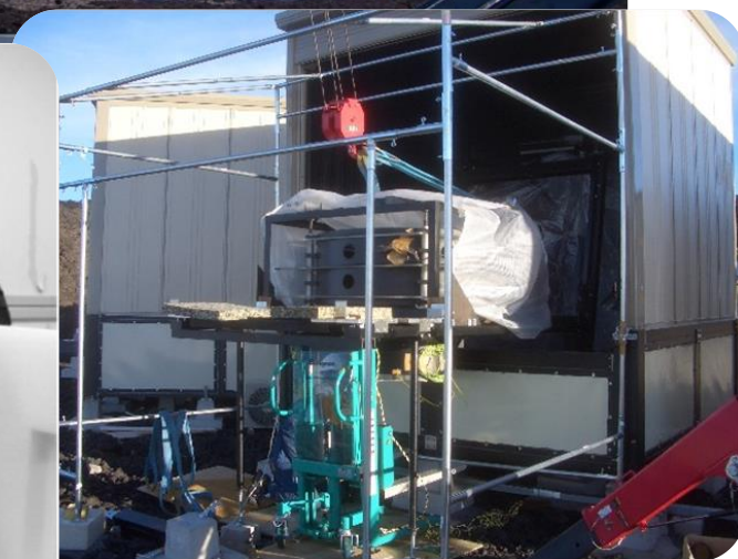
Installation of PLIs
