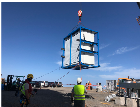
Figure 4: During the camera installation in September 2018
