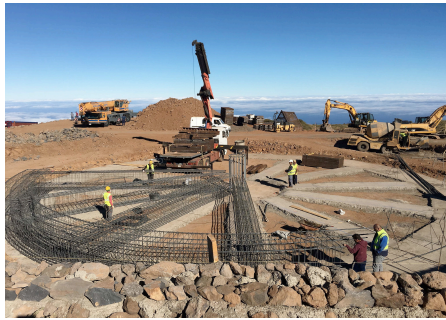
Figure 2: Building LST1 foundation
