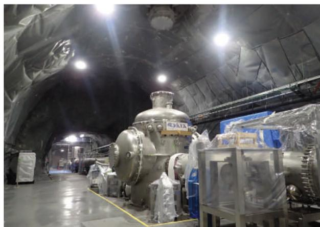
Fig. 4. Cryostat for the cryogenic mirror and the shaft for the vibration isolation system.
