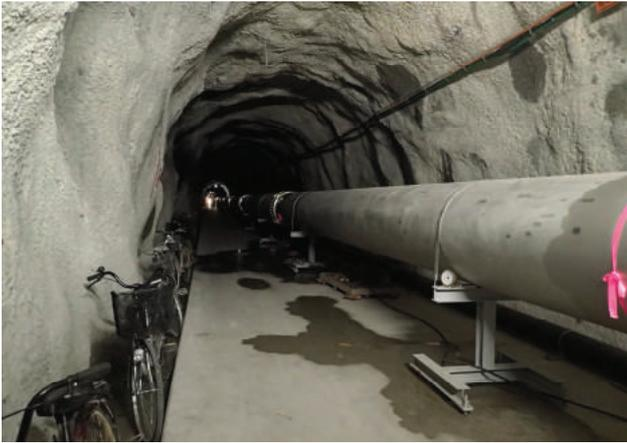
Fig. 6. 3-km beam tube in the Y-arm tunnel.
