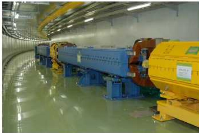
50 GeV Synchrotron Tunnel
