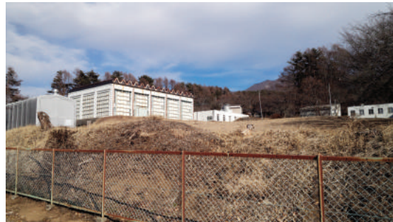
Fig. 5. The main site of the Akeno Observatory. There are the movable tent for a small atmospheric Cherenkov telescope, the large experimental hall, the research building and the lodging facility from the left.
