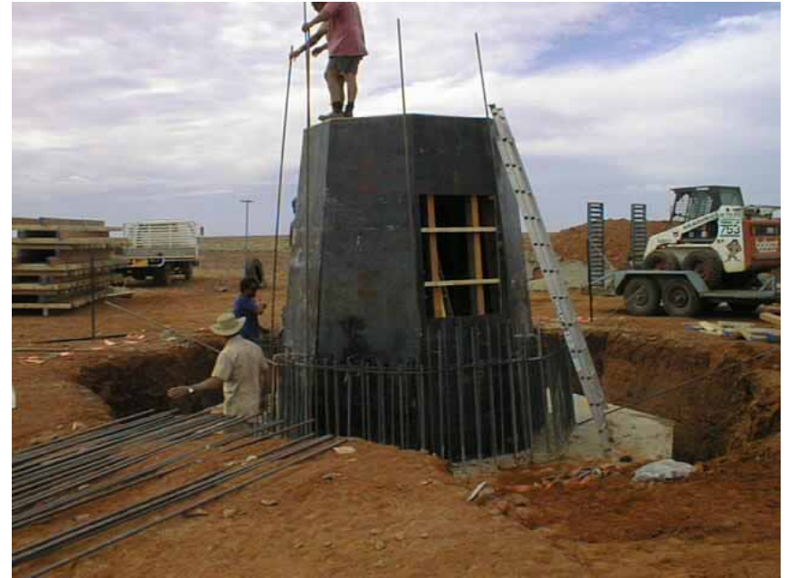
Formwork for the telescope pedestal base (Feb.'02)
