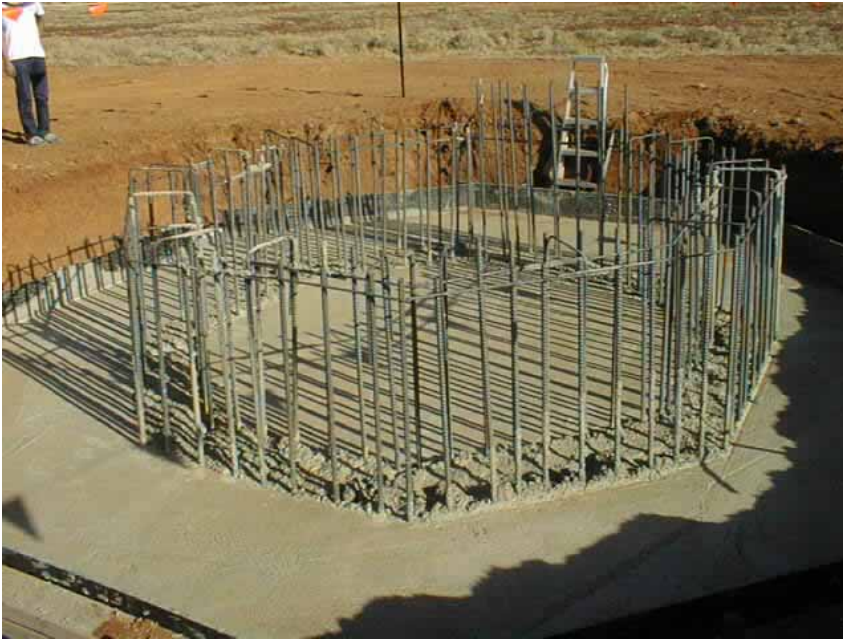
Construction of the telescope pedestal base (Jan.'02)
