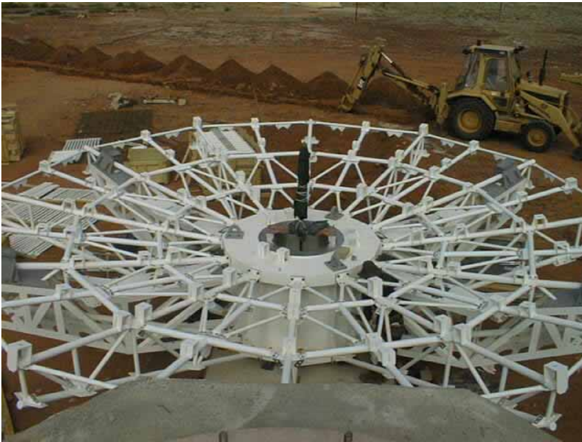
Assembly of the backing structure (Feb.'02)
