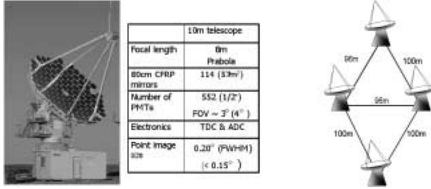
Figure 1: The 10 m telescope completed in February 2000 and the arrangement of CANGAROO-III four telescopes.
