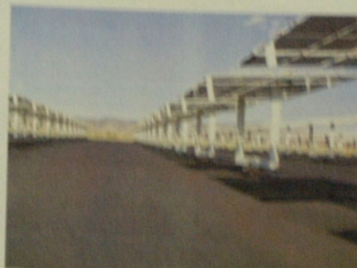
Blacktop sealant applied to reduce albedo from scattered light in the field
