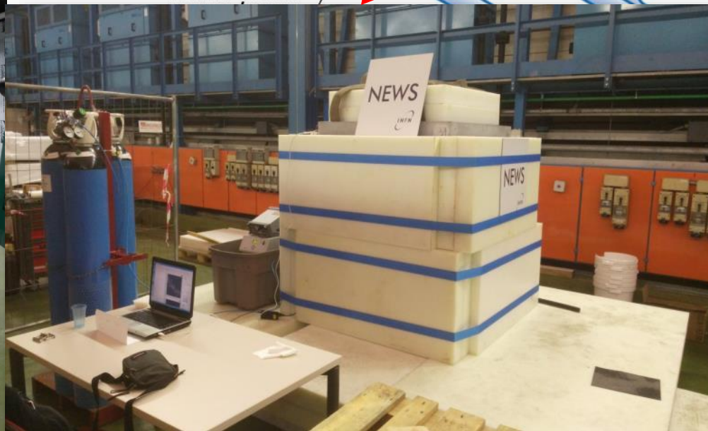
Part of Hall B for Detector Installation
