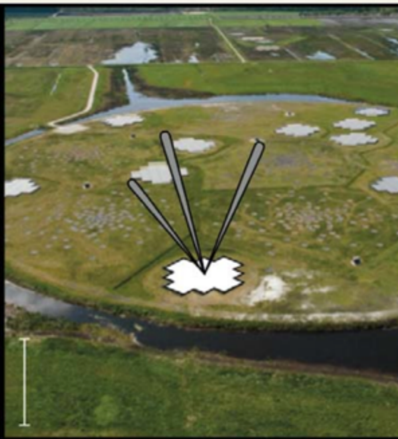
HBA station beam
